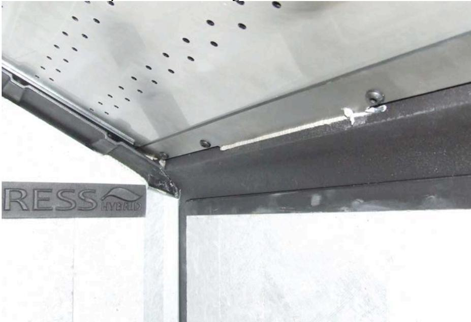
21. From the rear of the stove, cement in the gap around the entire secondary air inlet.
