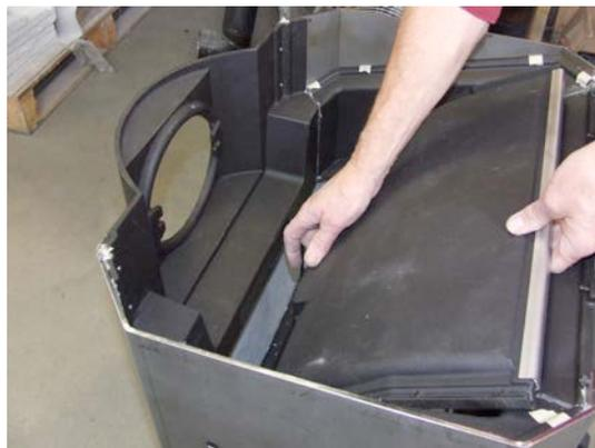
16. Pull the fireback assembly back out a bit and lay a line of furnace cement on the top of the air channels as shown below, then slide it back into place. Clean up excess cement.
