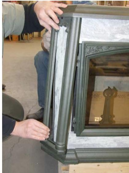
3. The tie rods are fastened with a 1/2" hex nut, which is located close to the leg bolts. Now lift upward on the large top frame just above the first of the cast corners and
