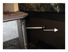
5. Lift up the bypass casting and rotate it 90° counter clockwise. Slide the stainless rod out of the flue collar and remove the bypass.
