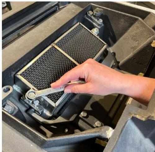
7. Lifting up and rotating 90 degrees, remove the original catalytic combustor through the open block-off collar. **Note:** your existing catalytic combustor may look different than your new one. Some older catalysts included two cast iron frames, top and bottom, which encased the catalytic element (constructed of either ceramic or steel material). Your new catalytic combustor will not utilize these frames and they may be discarded.
