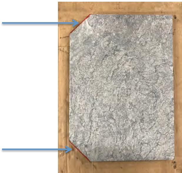
11. Pre cut (3) 1" lengths of gasket if replacing one stone panel, cut (6) 1" pieces you're replacing two. Place the stone retainer back on the stone. Push a 1" piece of gasket between the stone and retainer at each screw location and then start all the screws and star washers.
