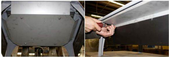
3. Locate the bolts under the front edge of the stove base that secure the andirons (follow the andiron down through the base of the stove). Loosen with a  $\frac{1}{2}$ " socket.
