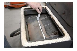
Replace the combustor shield, making sure the 2 round holes are toward the front of the stove and the "legs" fit in the notches on the flat flange of the combustor. Replace the top lid.
