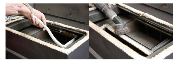
Squeeze a bead (about 1/8") of glue all round the gasket channel. Starting at the middle of the back, lay the gasket onto the glue, pushing back on itself lightly to help keep it "puffy". When you get all the way around, trim the gasket so the ends butt together.
