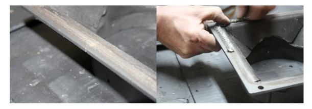
When you reach the starting point, cut the gasket so the ends butt together.
