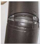
A fully locked connection at each joint is necessary to separate incoming air from exhaust
