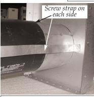
*Screw snorkel straps to the last piece of pipe and cut off excess*
