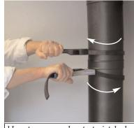
*Use strap wrenches to twist-lock pipe for a secure connection*
