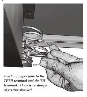
The problem could be a bad ON/OFF switch, a bad switch wire, or a faulty Transmitter. To narrow it down, start by disconnecting the Receiver box and reconnecting the lead from the ON/OFF switch. Turn on the stove with the switch. If the stove will not turn on with the switch, but worked with the jumper test, then it needs a new switch. If the switch works, but the Remote will not, then the problem is somewhere in the remote system.
