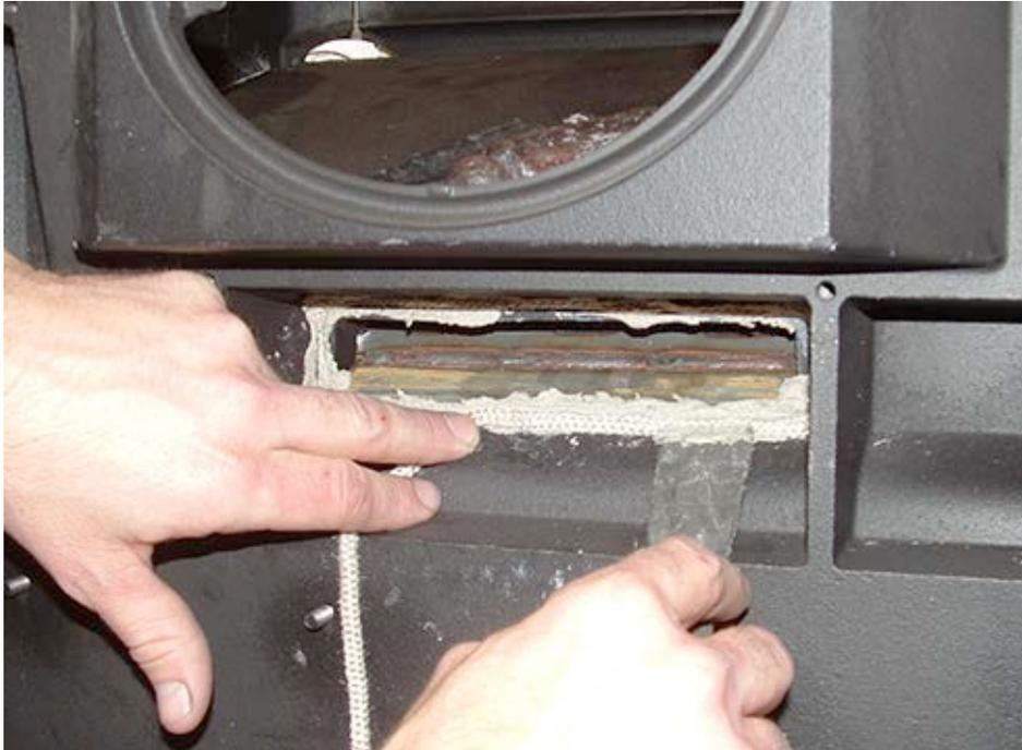
9. Starting on the inside right chamber of the fireback apply a generous amount of cement, do the same on the left side, then apply additional cement around the outer perimeter.
