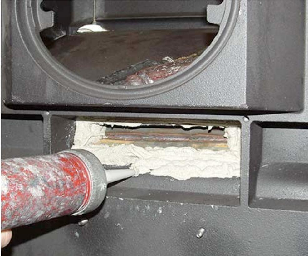
10. With wetted fingers smooth the cement, to help ensure a smooth airflow into the secondary fireback.
