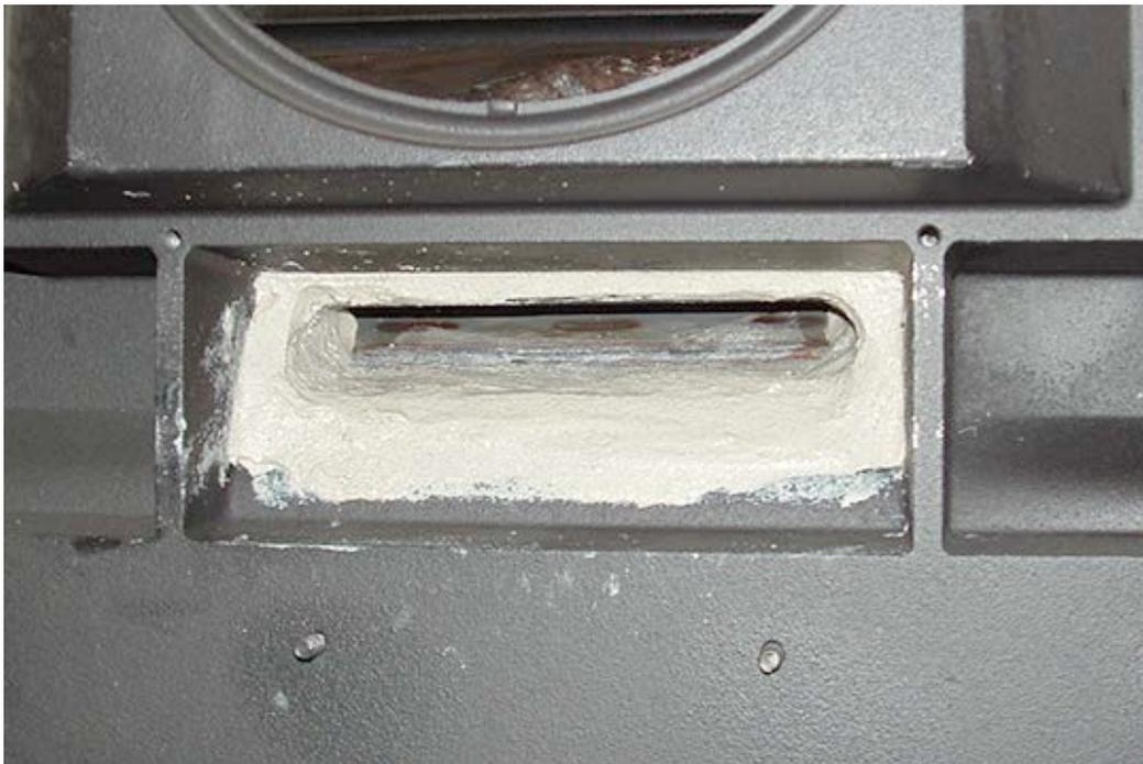
11. Through the loading door, apply cement along the bottom of the secondary fireback.
