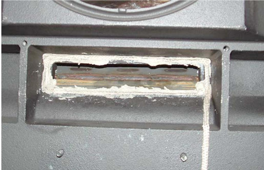
8. Take your cement and apply one more bead across the bottom edge, then tuck one more length of gasket into the bottom cement, tucking the gasket in with a putty knife. Cut any remaining gasket with scissors.
