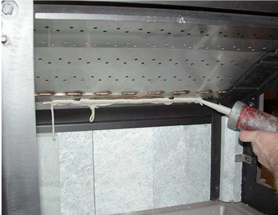
12. With wetted fingers smooth the cement pressing it into the area between the secondary fireback and cast iron frame.
