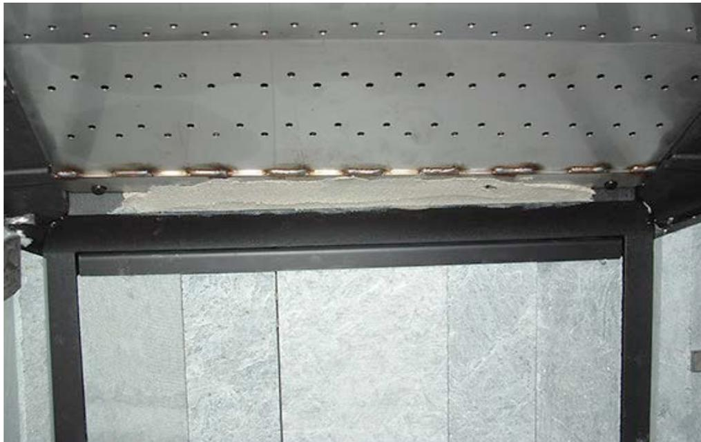
13. Apply a bead of the furnace cement to the back of the stove as shown in the photo below. The cement will make a seal between the back of the stove and the damper assembly.
