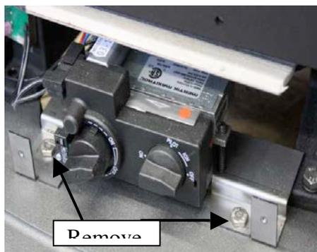
5. Use a 7/16" wrench to remove bolts that secure the control valve mounting plate to the base of the stove.
